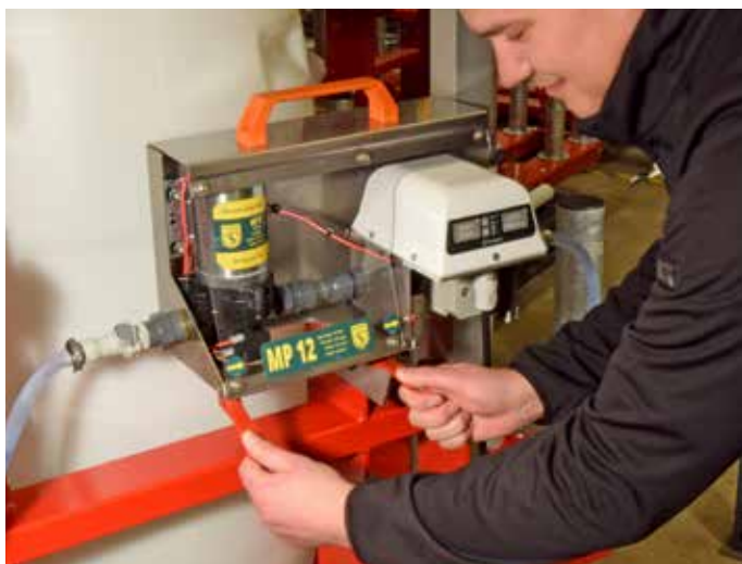
Figur 17 Hurtigfeste for enkel demontering.
